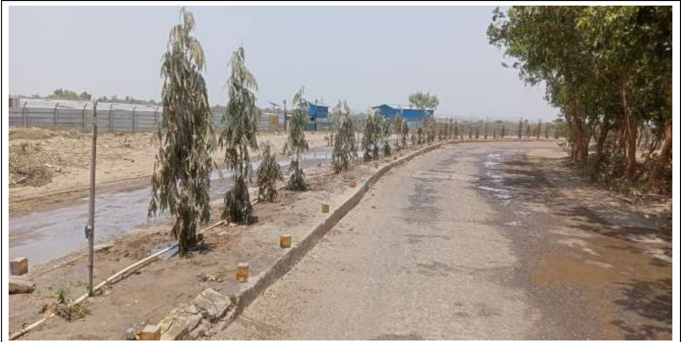
Water Sprinkling System along the Road
