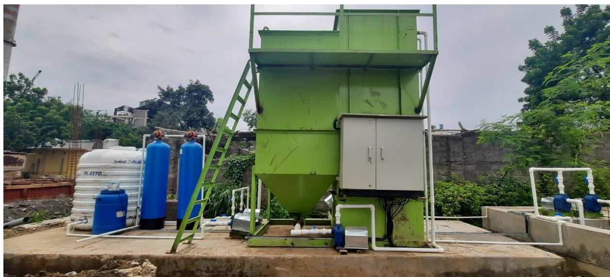
Sewage Treatment Plant Installed at Admine Building Main Gate (Capacity: 20 KLD)
