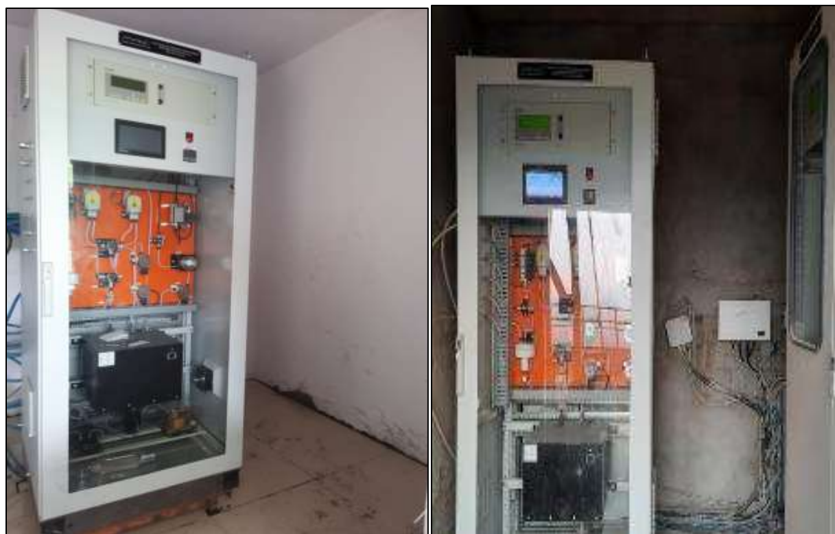
Installation of CEMS for Gaseous Emission Monitoring at Raw Mill + Kiln and CPP
